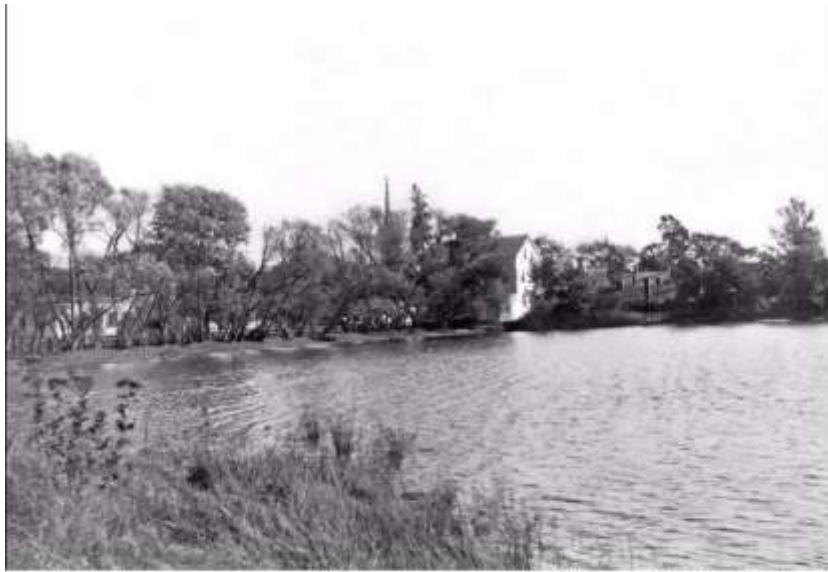
The Fulton's Pond site was once owned by Robert MacMoran and his son-in-law Robert Fulton who erected a factory that produced a variety of knives.
