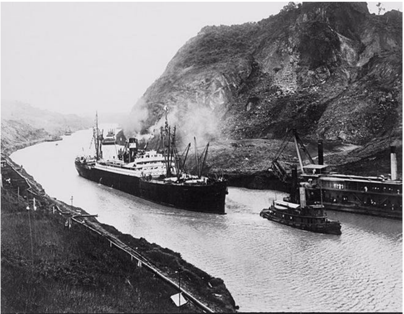
Panama Line steamer USS Ancon enters the Panama Canal in August 1914.
