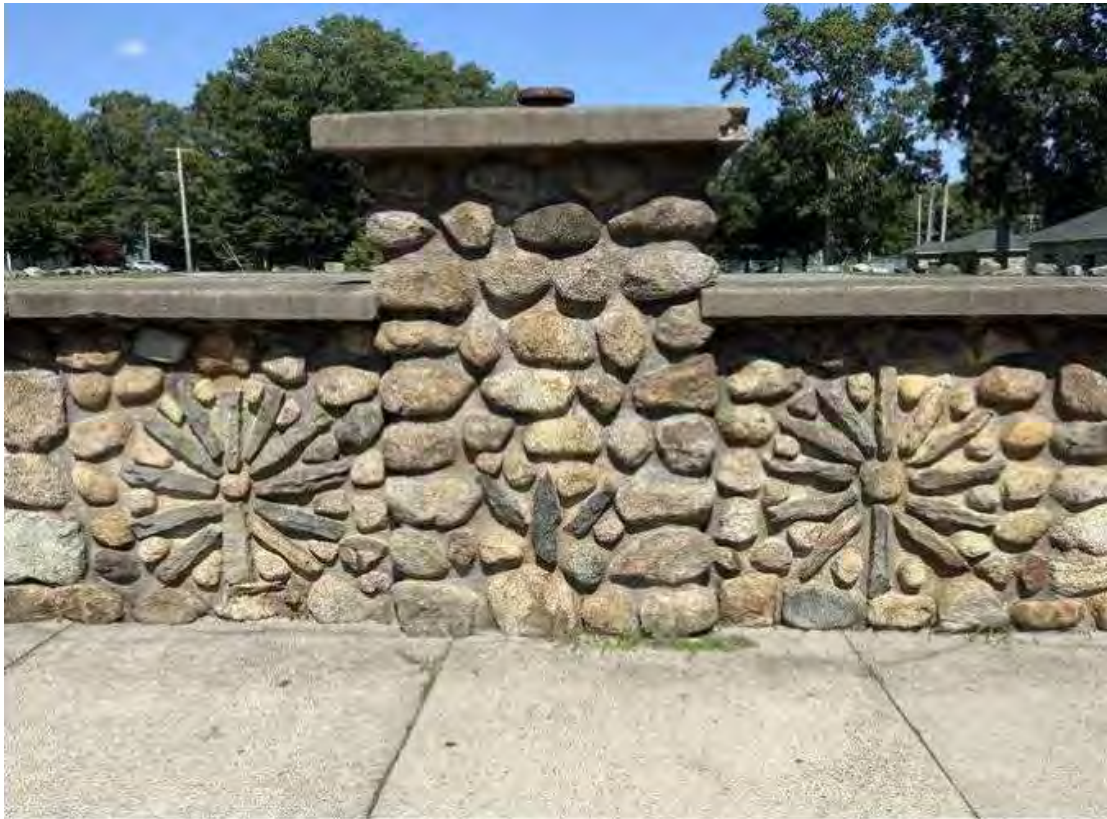
One of the most enduring features of Memorial Park is the pair of four-foot walls that curve at the entrance to Hope Street. About every 10 feet the masons added a design that some said resembled the limbs of a tree branching out from a trunk. The long stone wall entrance remains an enduring Mansfield landmark.
